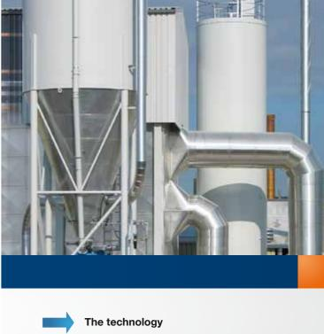
The necessary absorption material is fed to the flue gas flow using a feeding system. The reaction product is then separated in an hose filter plant and removed.
